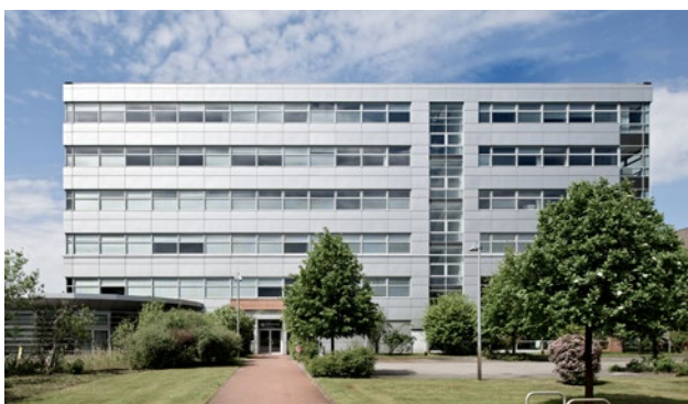
Berlin, Büro, Archiv, Refurbishment Bestand, 125 Mio. Euro
